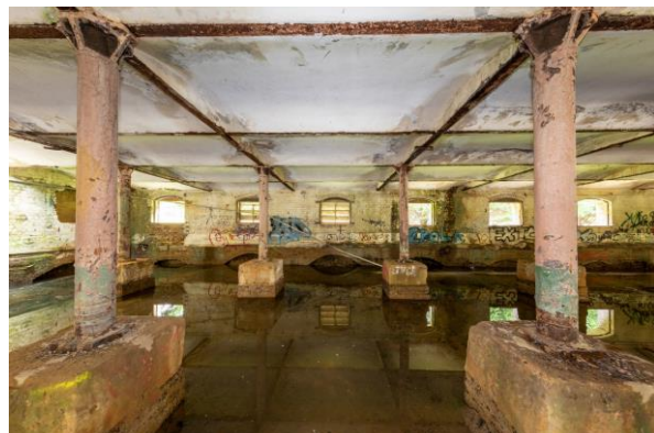
Figure 7 The vaulted concrete soffit, cast iron columns and sandstone/concrete/brick footings at the undercroft of the M1 machine room.
